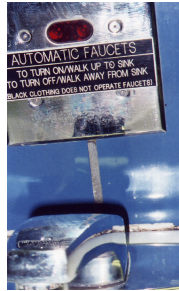
Figure 1.10 A sign in the restrooms at Cincinnati airport. Because it is not visible to the user as to what to do to turn the faucet back on and off, a sign has been added to explain what is normally an everyday and well-learned activity. It does not explain, however, what to do if you are wearing black clothing.
